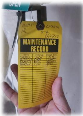
Backflow testing tag
